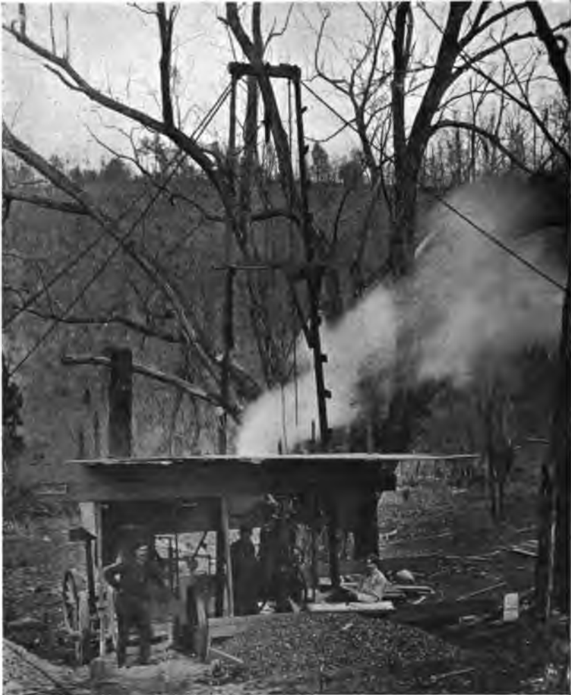
PLATE 18.—Sullivan Hydraulic Diamond Drilling Rig at Shaft 8, Rondout Siphon.
